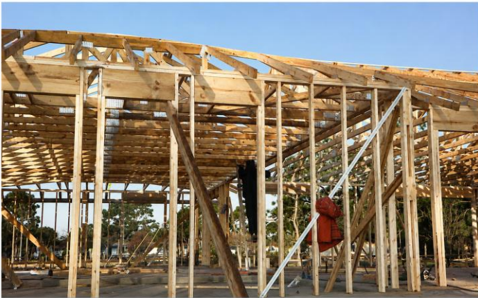
Miller Lane Under Construction
